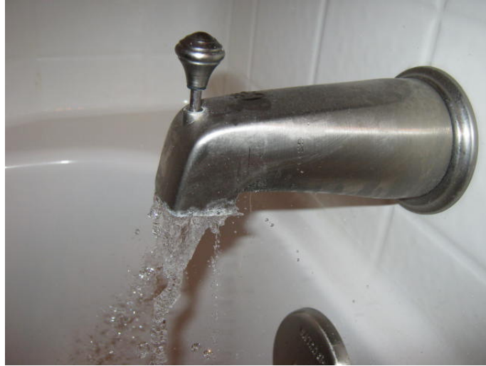
The shower diverter leaks
