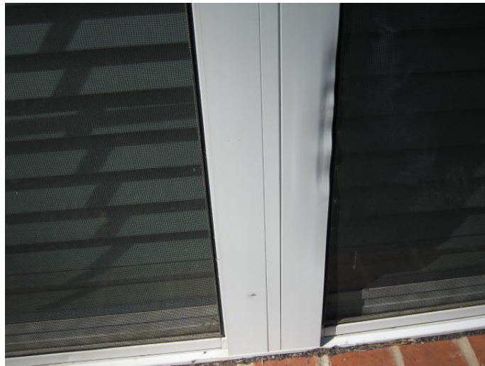
Window at the left side has a damaged frame (this is cosmetic only)
