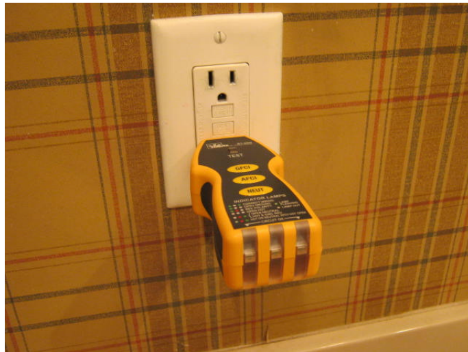
Receptacle outlet was not functional and should be repaired.
